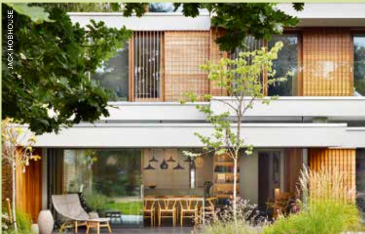
The designers at Coupdeville Architects incorporated timber louvres to provide this contemporary dwelling in west London with shade and privacy
